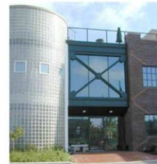
Architectural metal, brick and glass block invoke an industrial character.
