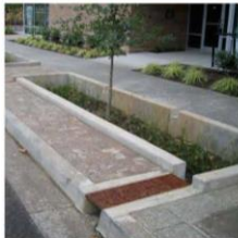
Stormwater management integrated in streetscape design.
